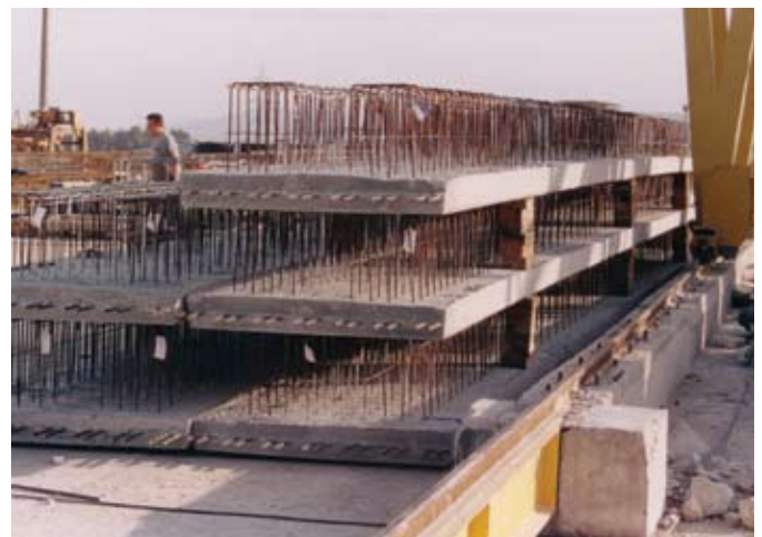
Fig. 2: Prestressed precast slabs at a casting yard in Spain
