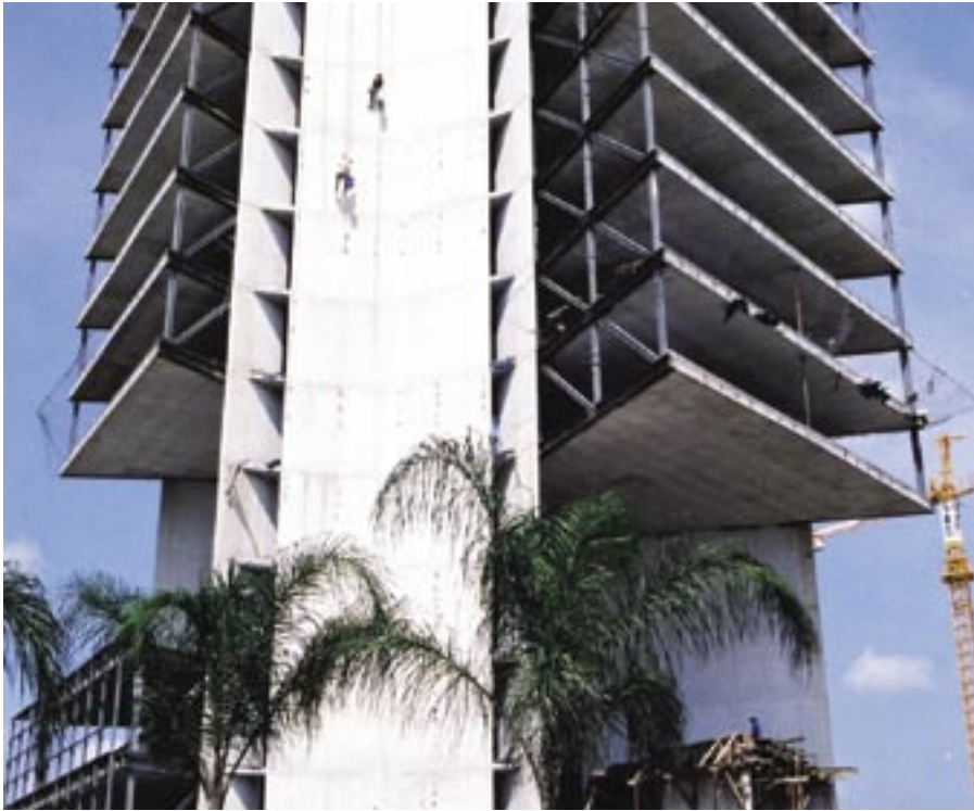
Fig. 1: Office modules jut out from the curved central cores constructed of white concrete, giving the tower a light, airy feel
