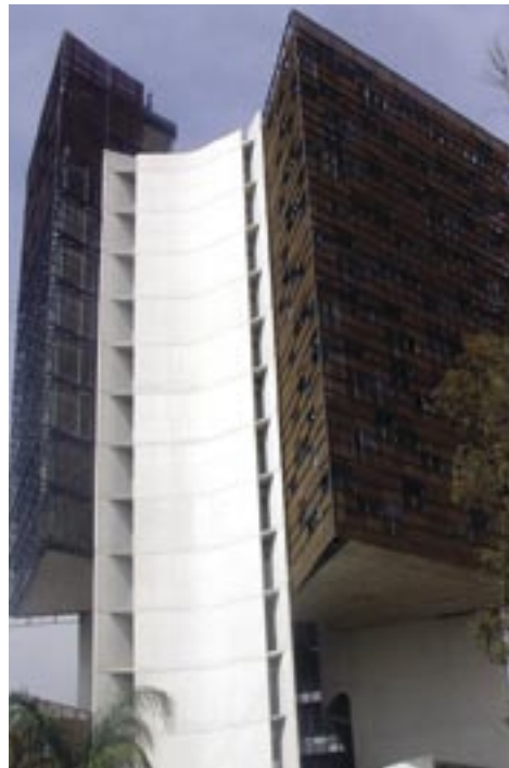
The CUBE tower in Zapopan, near Guadalajara, Mexico. The building is located in a high profile area with a highly competitive market for office space. Thus, the clients stressed the need for singularity
