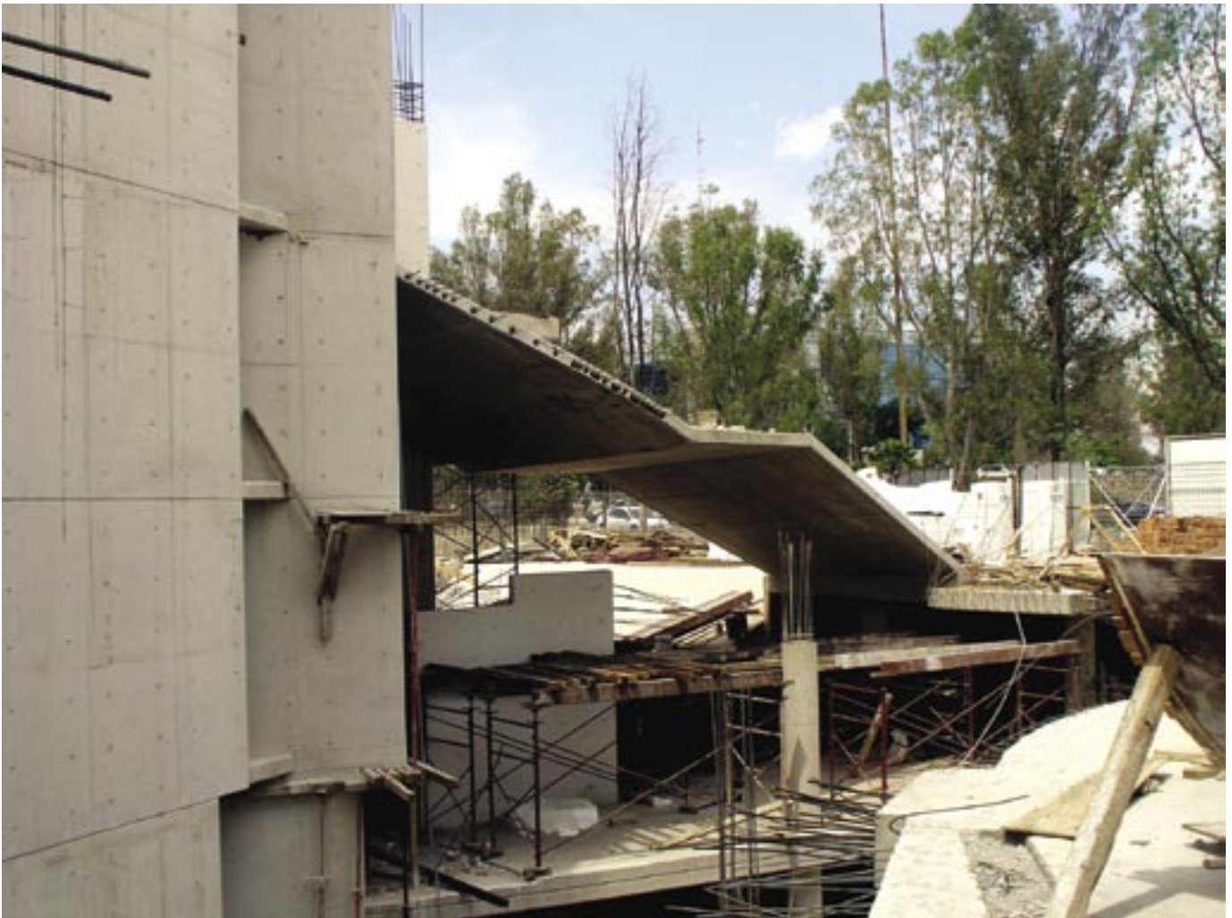
Fig. 7: The slender main stairway, leading to the reception area, under construction
