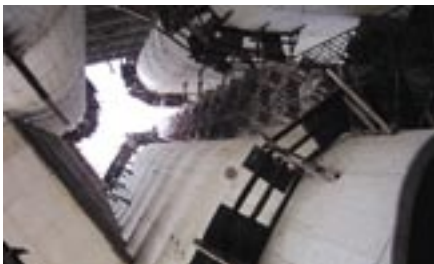
Fig. 1: Office modules jut out from the curved central cores constructed of white concrete, giving the tower a light, airy feel
