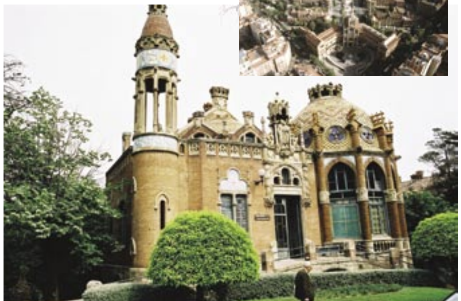
Fig. 1: One of the many Art Nouveau-style buildings comprising the Sant Pau Hospital (inset: overall view of the existing hospital with a superimposed rendering of the new construction)
